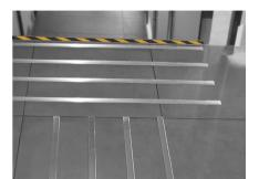
**Novoband Access** is a profile made of natural aluminum designed to be installed as an element of guidance for people with visual disabilities within the EMAC®'s Universal Accessibility and Safety System. This profile
