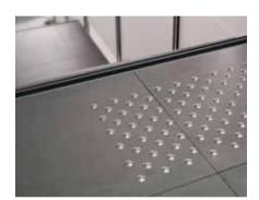
The **Novotop Access aluminum** tactile nails provide a warning solution to identify areas with obstacles, or areas where there is a change of level or an unprotected gap, such as staircases and open platforms.
